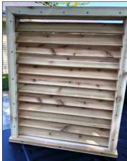
One of the louvers before it was mounted in the structure.
