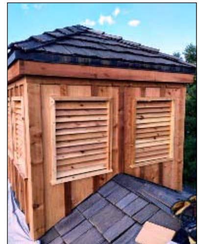
Shutters on the completed cupola and mounted on the building roof.
